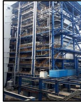
Gambar 2. Circulating Fluidized Boiler
